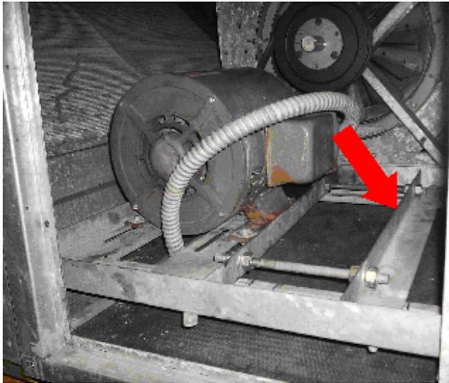
When the new parts arrived, the sheaves were replaced and the belts installed. Applying knowledge from a recent NAVSEA training class on Belt-driven equipment maintenance, it was determined that the belt size did not match the sheave size. While new B-size belts needed to be ordered to match the B-pitch of the sheaves, the unit needed to be returned to service in the meantime. The team worked together to align and tension the belts. Using a
